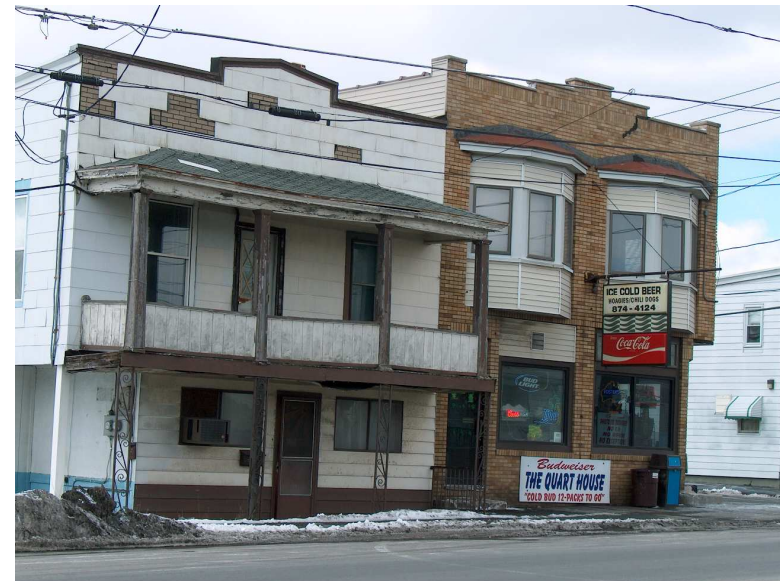
These roofs are not visible
