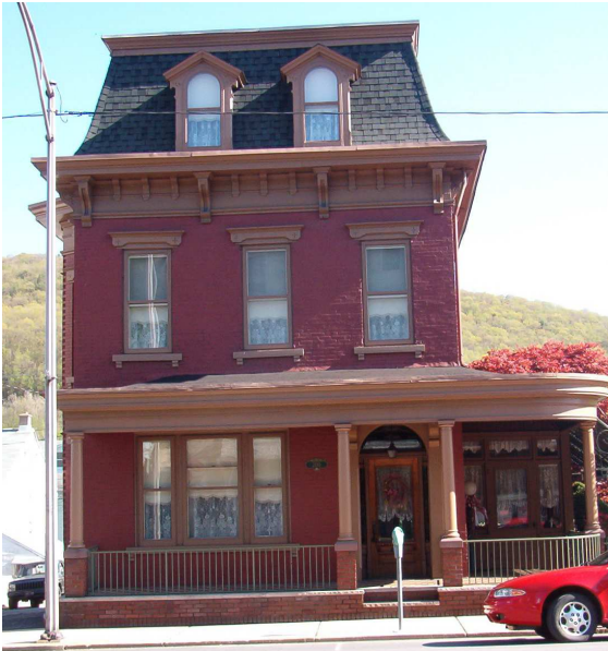
This roof is visible
